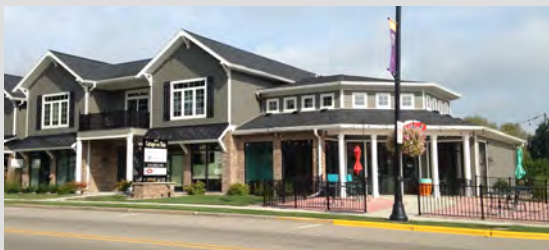
Mixed use developments provide two or more uses either on a single tract of land (i.e., horizontal mixed use - see below), or within a single building (i.e., vertical mixed use). Typically the first floor is retail, but office or a public use may also occupy the first floor.
