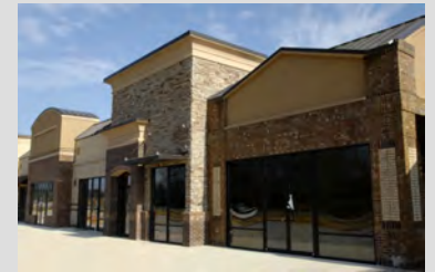
Desired design for a retail building. The color palette includes natural and earth tones. Building uses brick (primary) and EIFS (secondary), and architectural details that breakdown the facade to human scale. There are varying building planes and heights.
