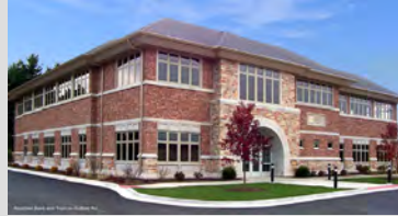
Left, retail building with primary facade using fiber cement siding with stone as an accent material. Right, retail building with primary facade using stone and brick with EIFS as an accent material. Both meeting a desired natural color palette.
